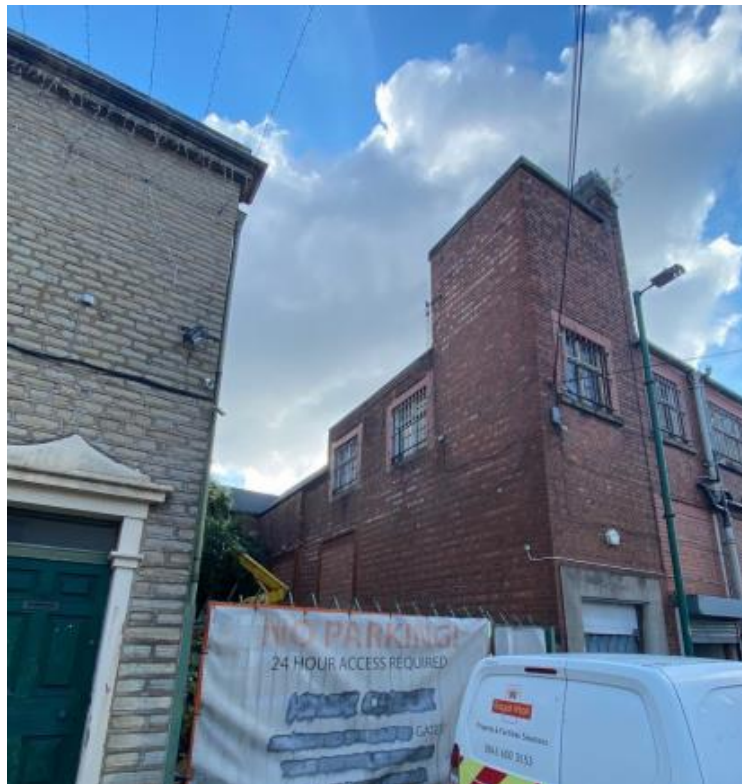
Photo 6: Side Elvation from Hamnett Street
